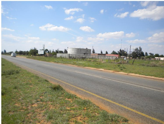
Sebayeng-Dikgale Regional Water Scheme: Reservoir
