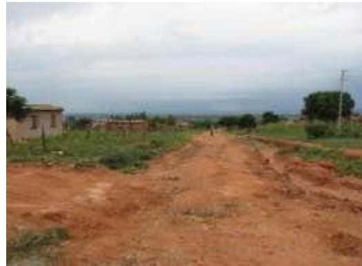
Figure 4: Erosion due to Lack of Stormwater Infrastructure road infrastructure
