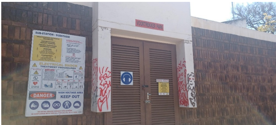
Diagram 184: Voortrekker Park substation to the east of the CBD
