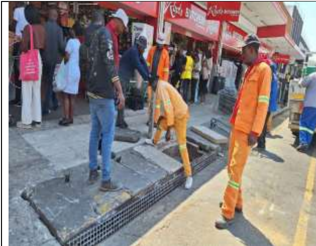
Unblocking of Storm Water Drainage System in the City CBD
