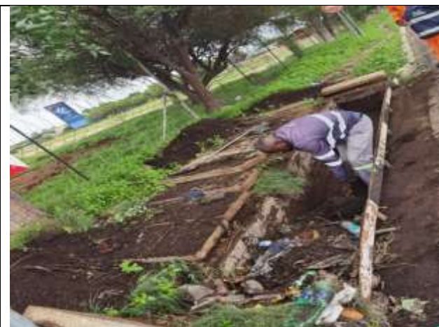
Unblocking Storm water Drainage System
