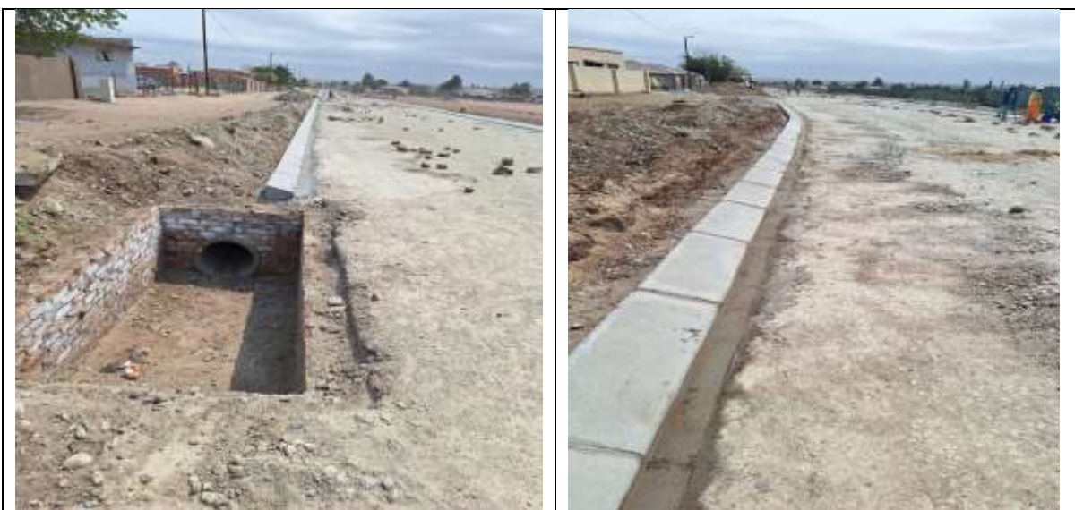
Paving of internal Streets at Seshego Zone 6
