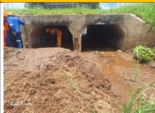
Unblocking Storm water Drainage System
