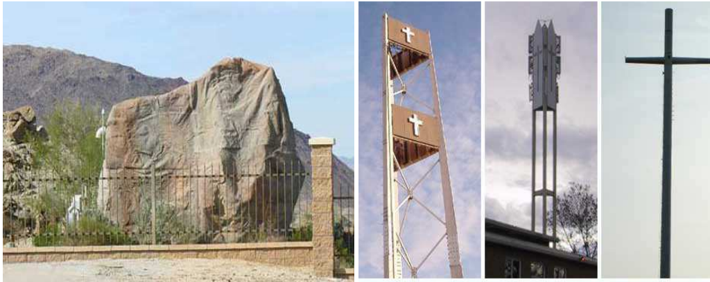
ECF designed as an architectural feature
