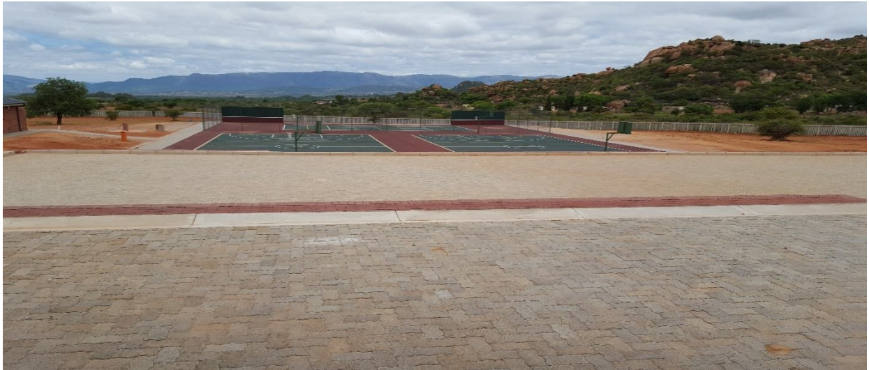
Ga-Molepo Sports Complex constructed at Ga-Molepo
