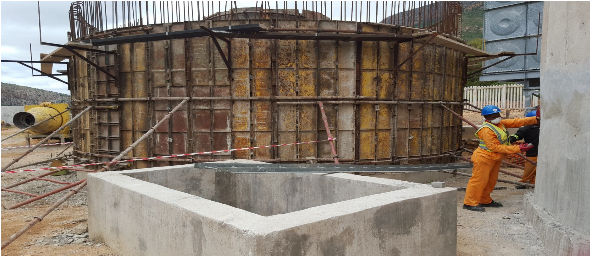
Chuene/Maja Regional Water Scheme under construction at Ga-Chuene
