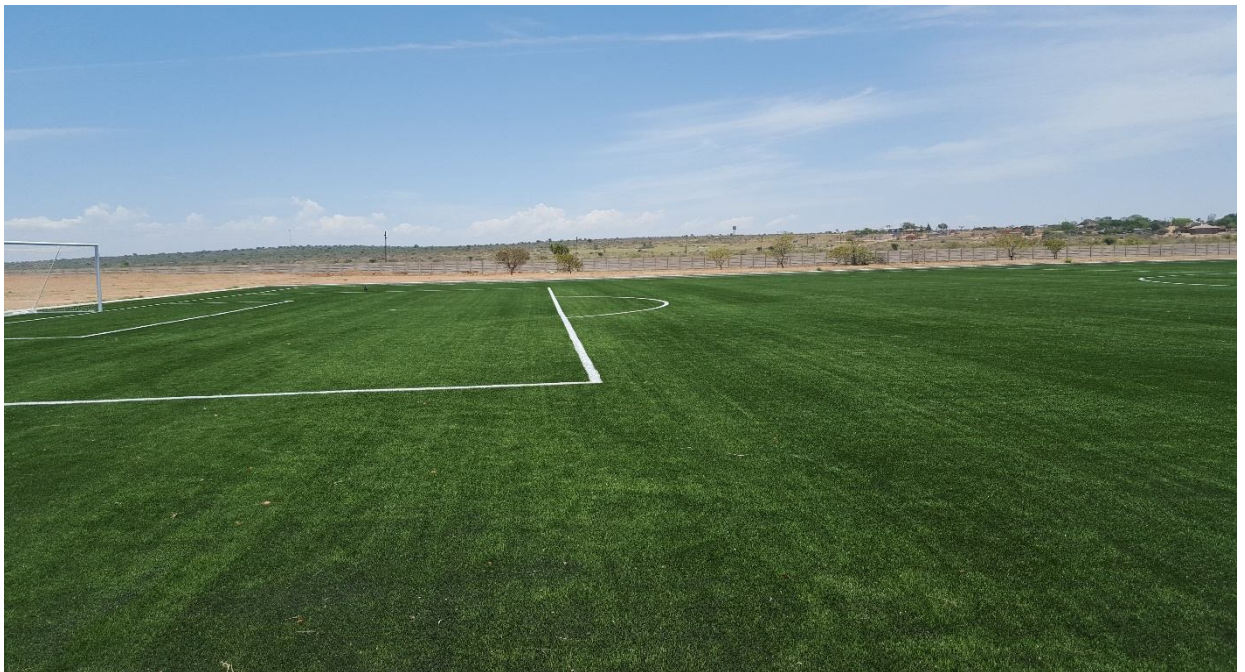
Ga-Manamela Sports Complex constructed at Ga-Manamela
