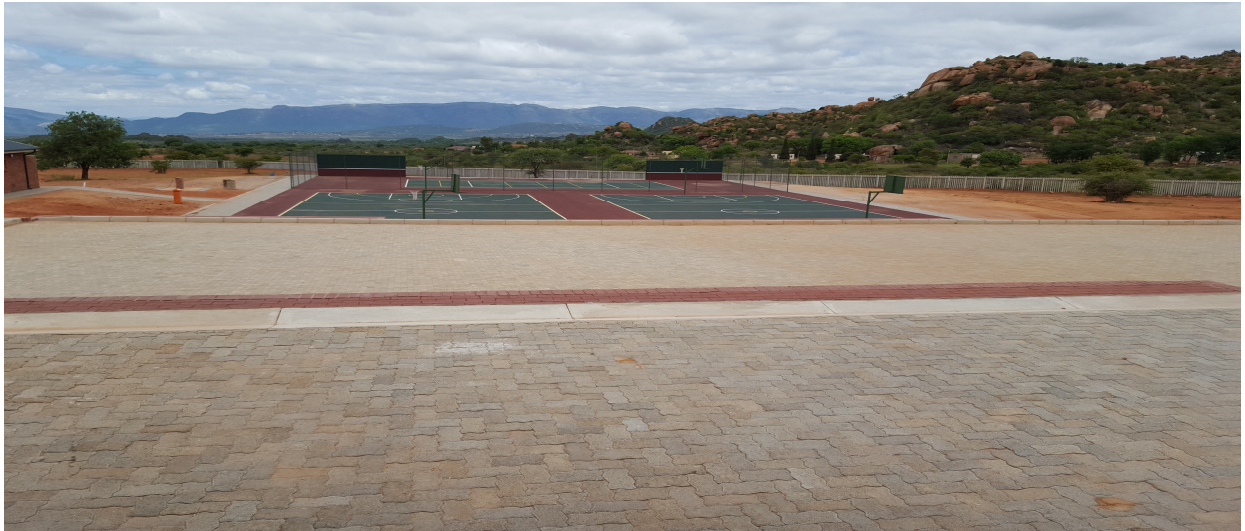
Ga-Molepo Sports Complex constructed at Ga-Molepo
