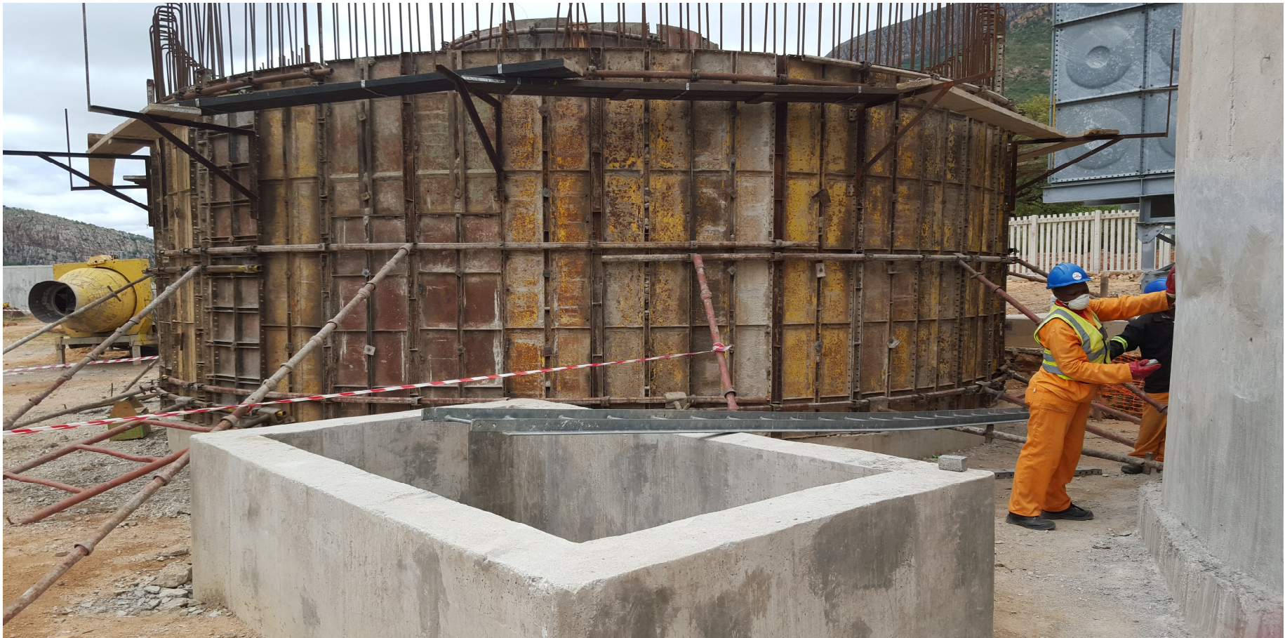
Chuene/Maja Regional Water Scheme under construction at Ga-Chuene
