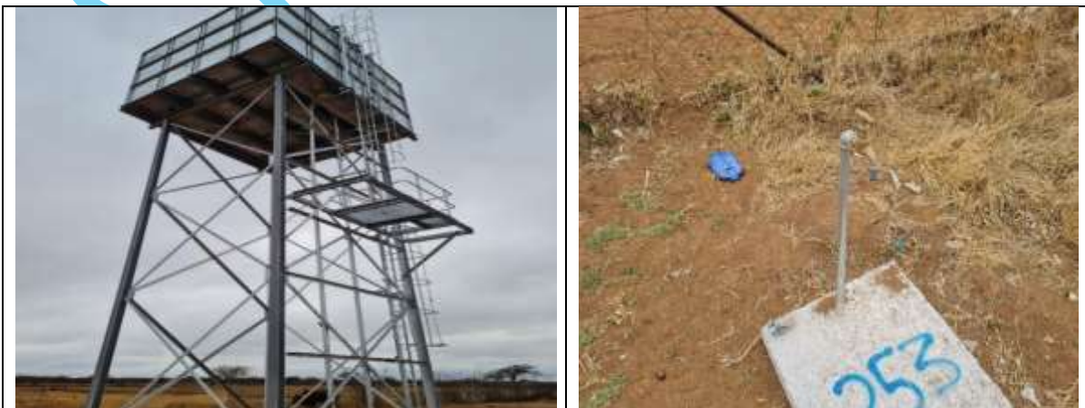
Progress Photos 1 -Aganang RWS (Ramalapa,Mashamaite,Makgodu,Mars)-Steel tank and stand pipes 1
