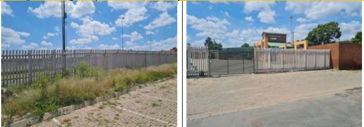
Fencing of Itsoseng Entrepreneurial Centre Completed 3
