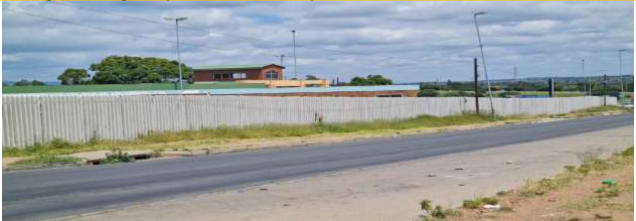
Fencing of Itsoseng Entrepreneurial Centre Completed 2
