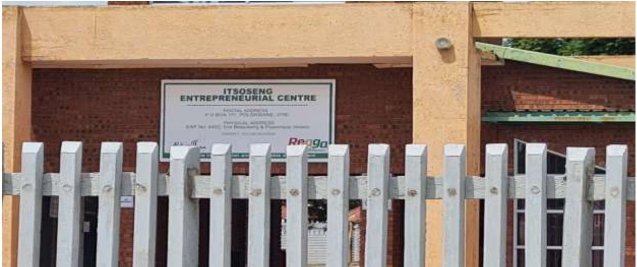
Fencing of Itsoseng Entrepreneurial Centre Completed 1
