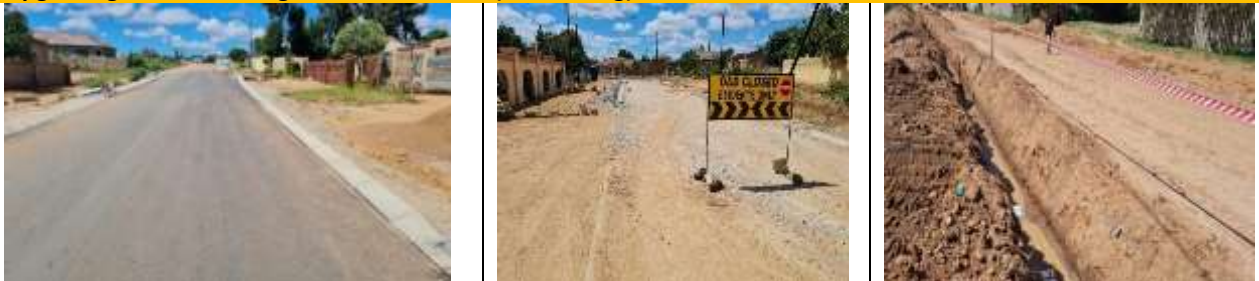
Upgrading of internal ring Road in Toronto (Mankweng)
