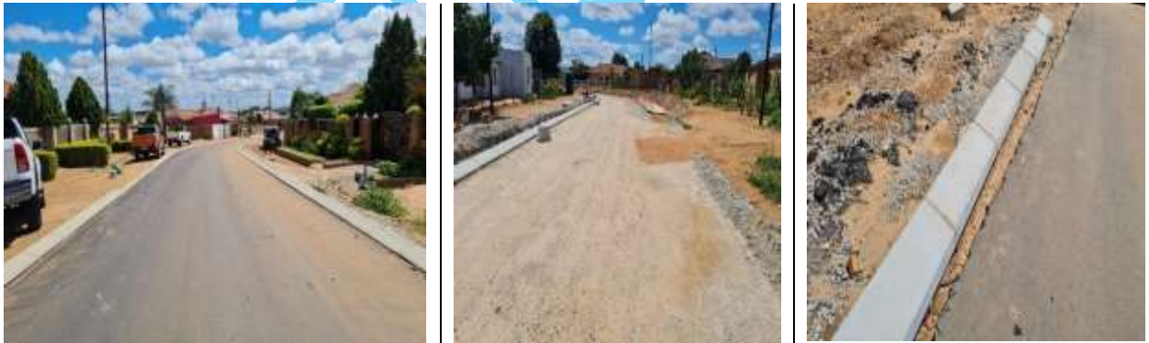
Upgrading of internal ring Road in Toronto (Mankweng)
