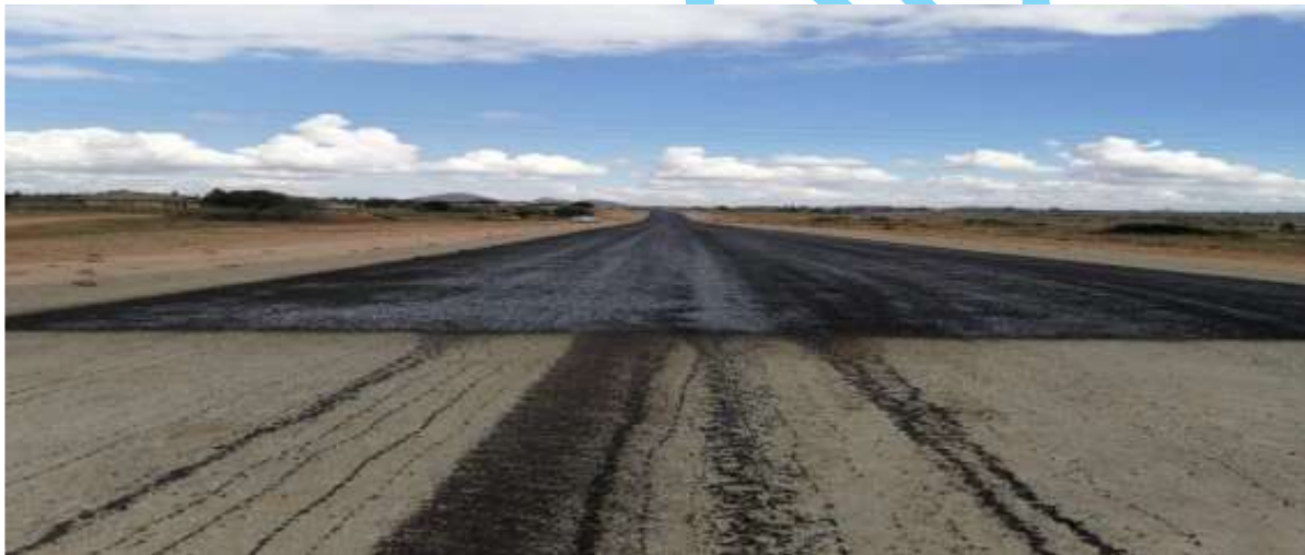
Upgrading of road from Mohlolong to Kalkspruit
