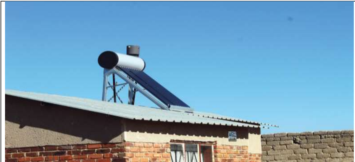
Solar geysers Installed at Seshego's Ext 71 and 75
