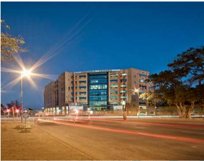
Buildings within City of Polokwane CBD 1
