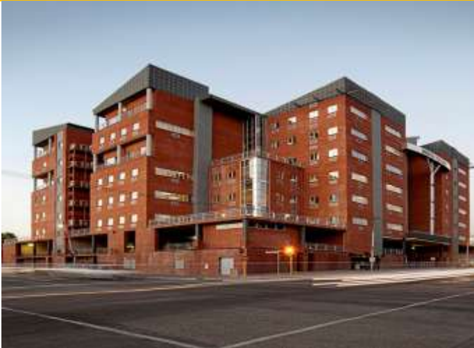
Buildings within City of Polokwane CBD 2
