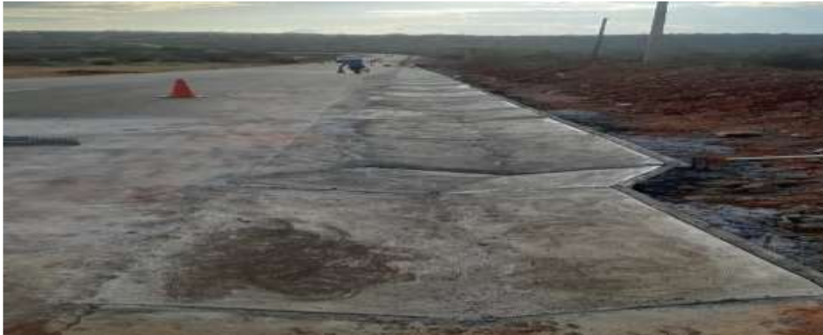
Upgrading of Arterial road in Ga Rampheri
