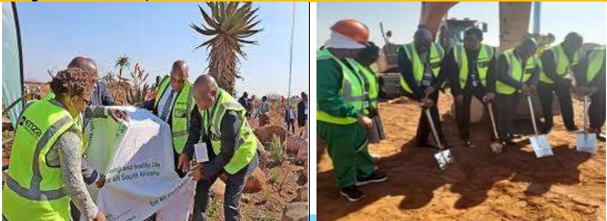
Health Minister, Dr Joe Phaahla, and other government officials turned the first sod to mark the birth of the groundbreaking new Limpopo Central Hospital
