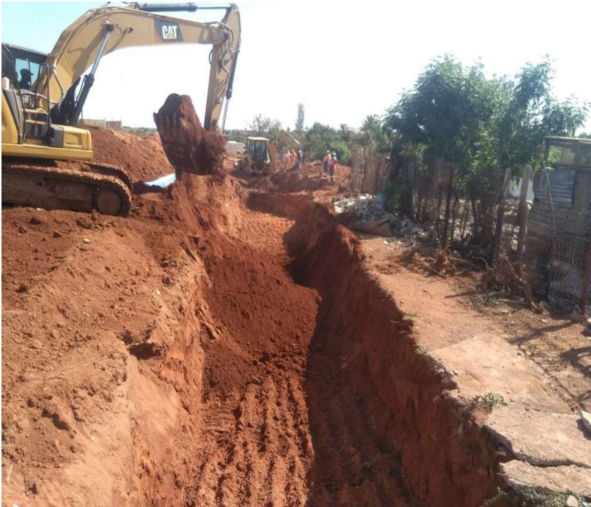
Excavations of trenches and preparation for laying of pipes in a village.
