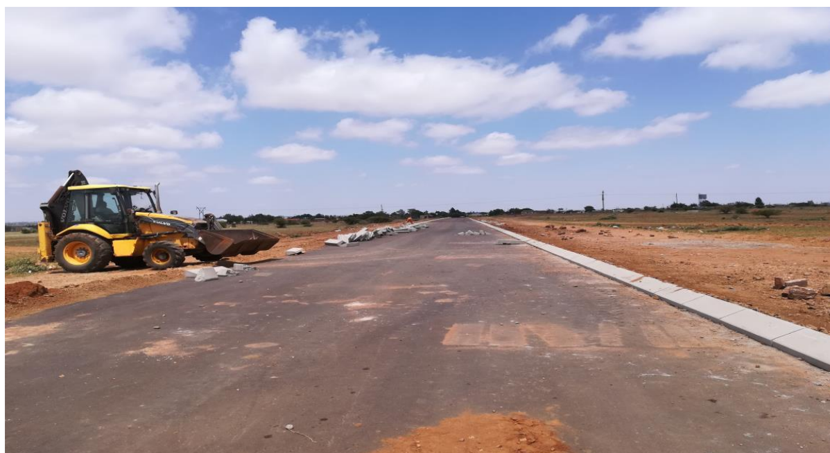
Ring road connecting Ga Hlahla to Ga –Semenya Villages. 3.5 km long
