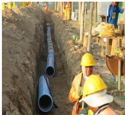
Pipe laying in Seshego
