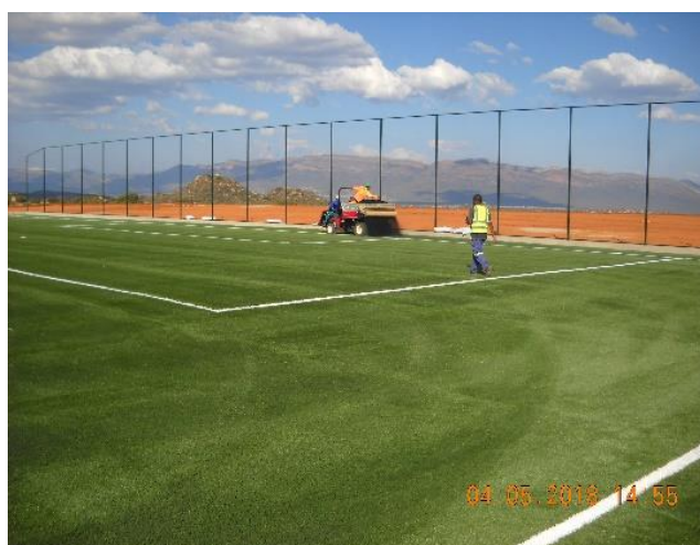
Construction of soccer pitch at Molepo stadium
