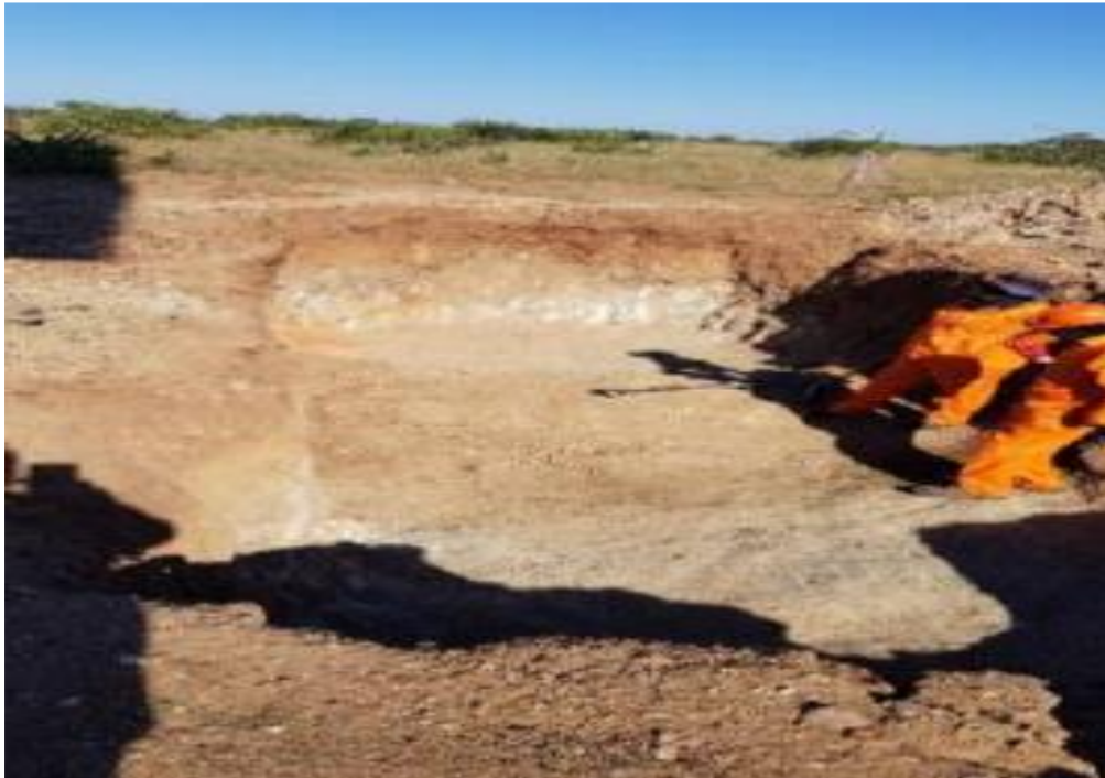
Epwp workers engaged on water project in excavation of footing
