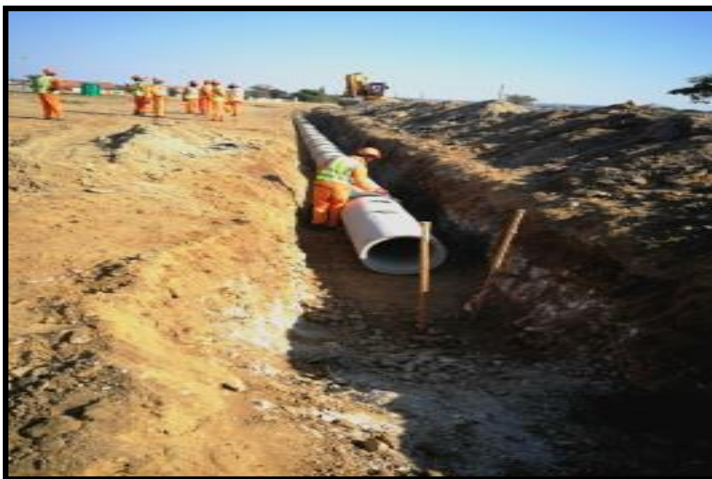
Epwp workers engaged on a road project installing storm water culverts
