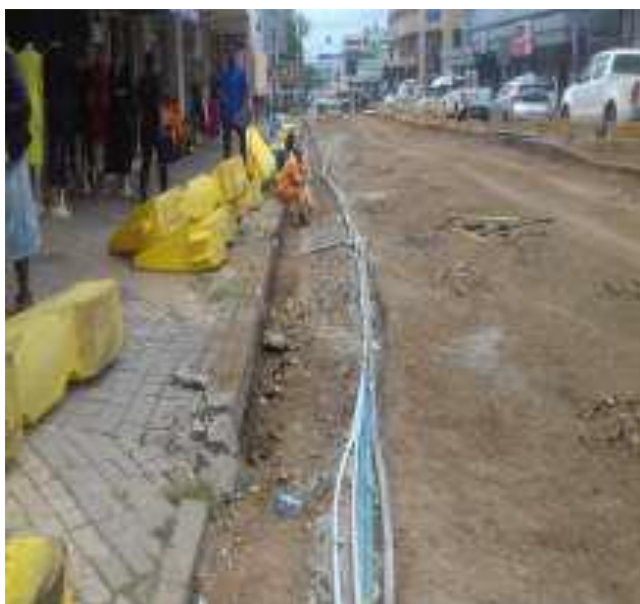
Rehabilitation of Thabo Mbeki Street in the CBD depicting relocation of underground telecommunications infrastructure
