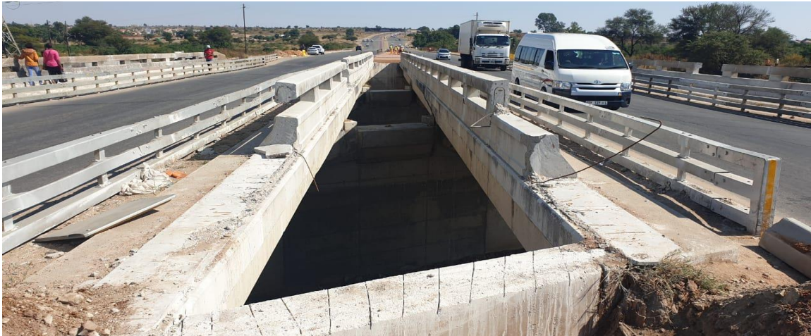
Widening of the sand river bridge project
