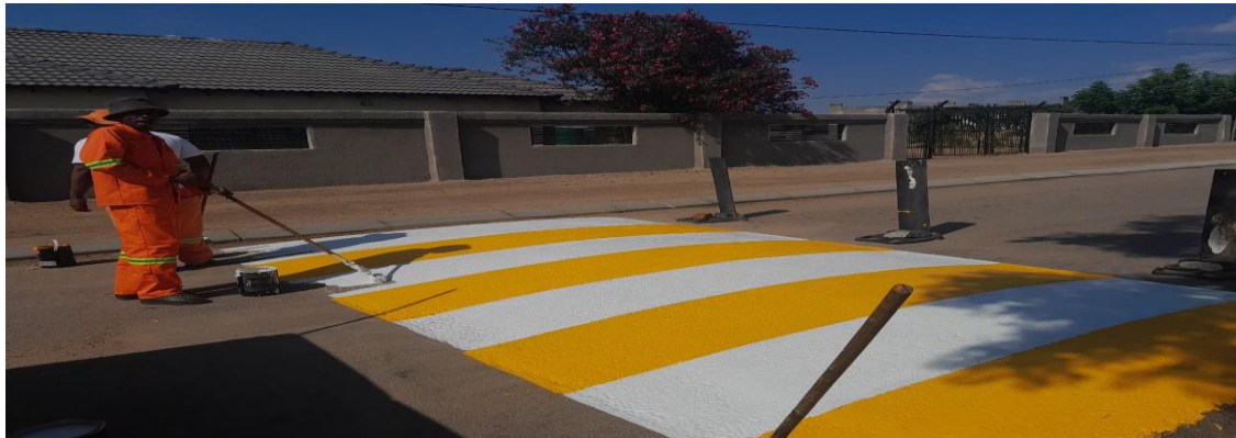
Routine maintenance (Speed hump marking)
