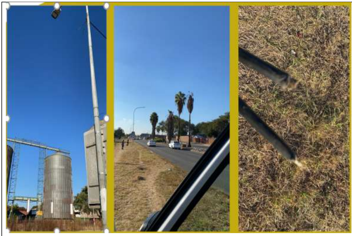
Figure: Damage and repair process of fiber connection.
