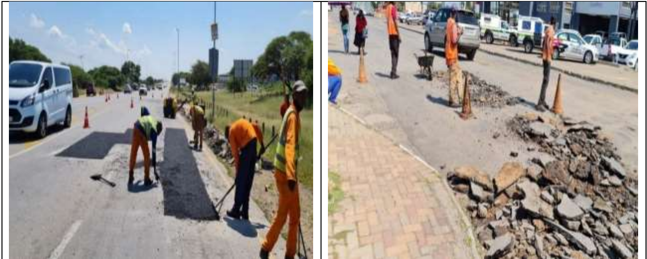
Potholes Repairs in the City CBD (2021)
