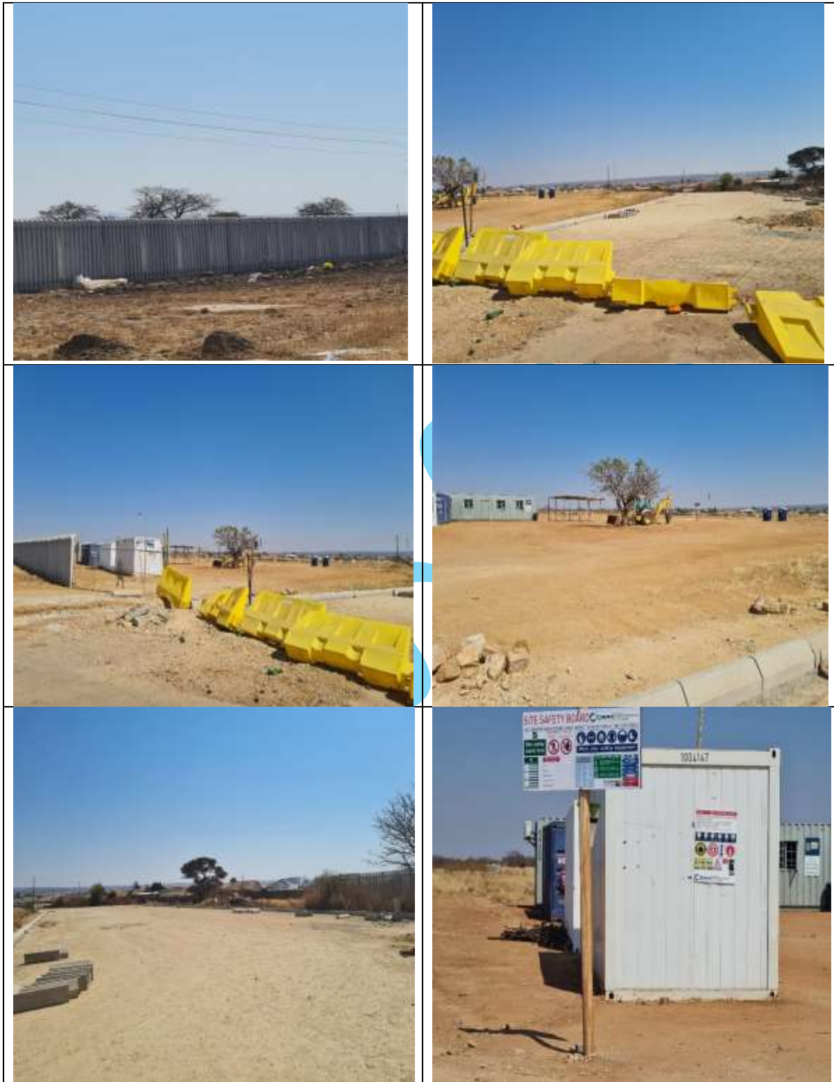
Construction of the Bus Depot at Seshego as at 10 August 2021
