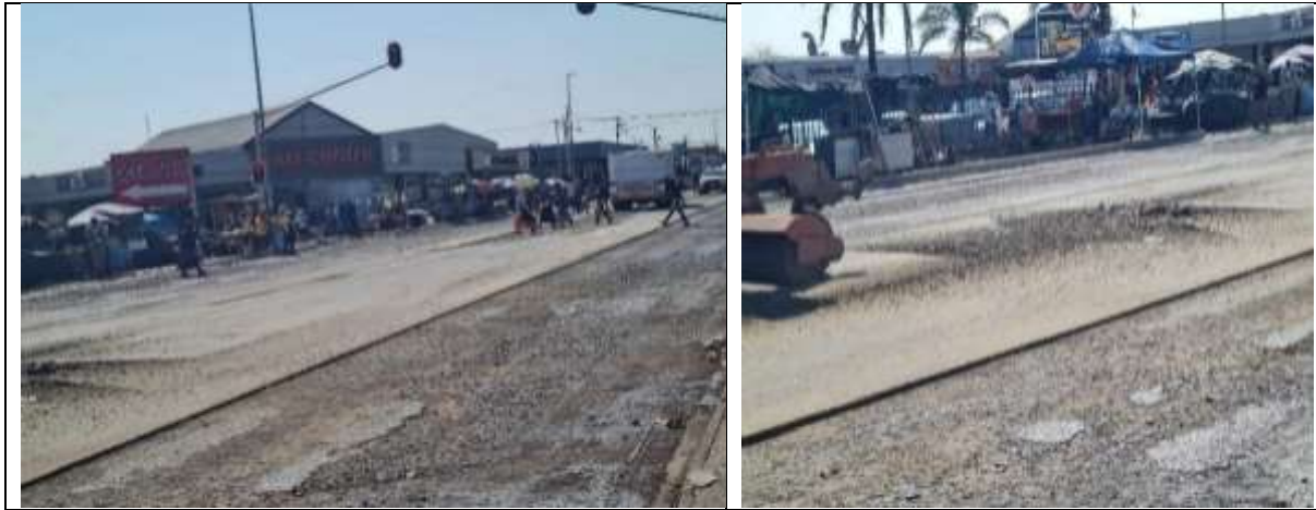
Rehabilitation of City CBD Roads as at 01 September 2021
