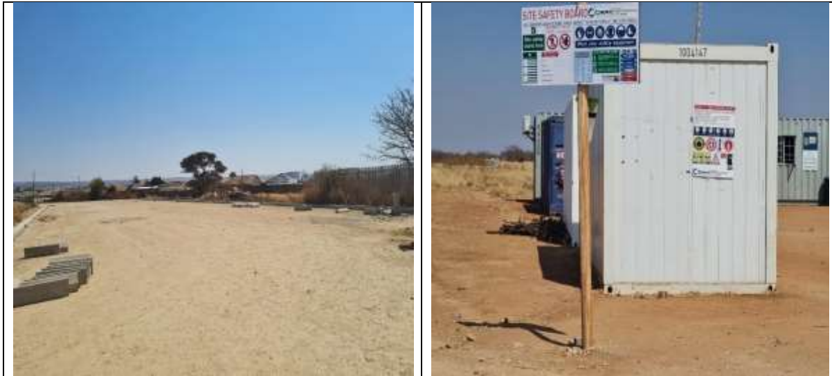
Construction of the Bus Depot at Seshego as at 10 August 2021
