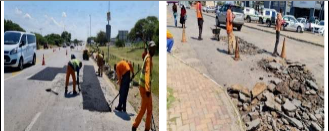
Potholes Repairs in the City CBD (2021)
