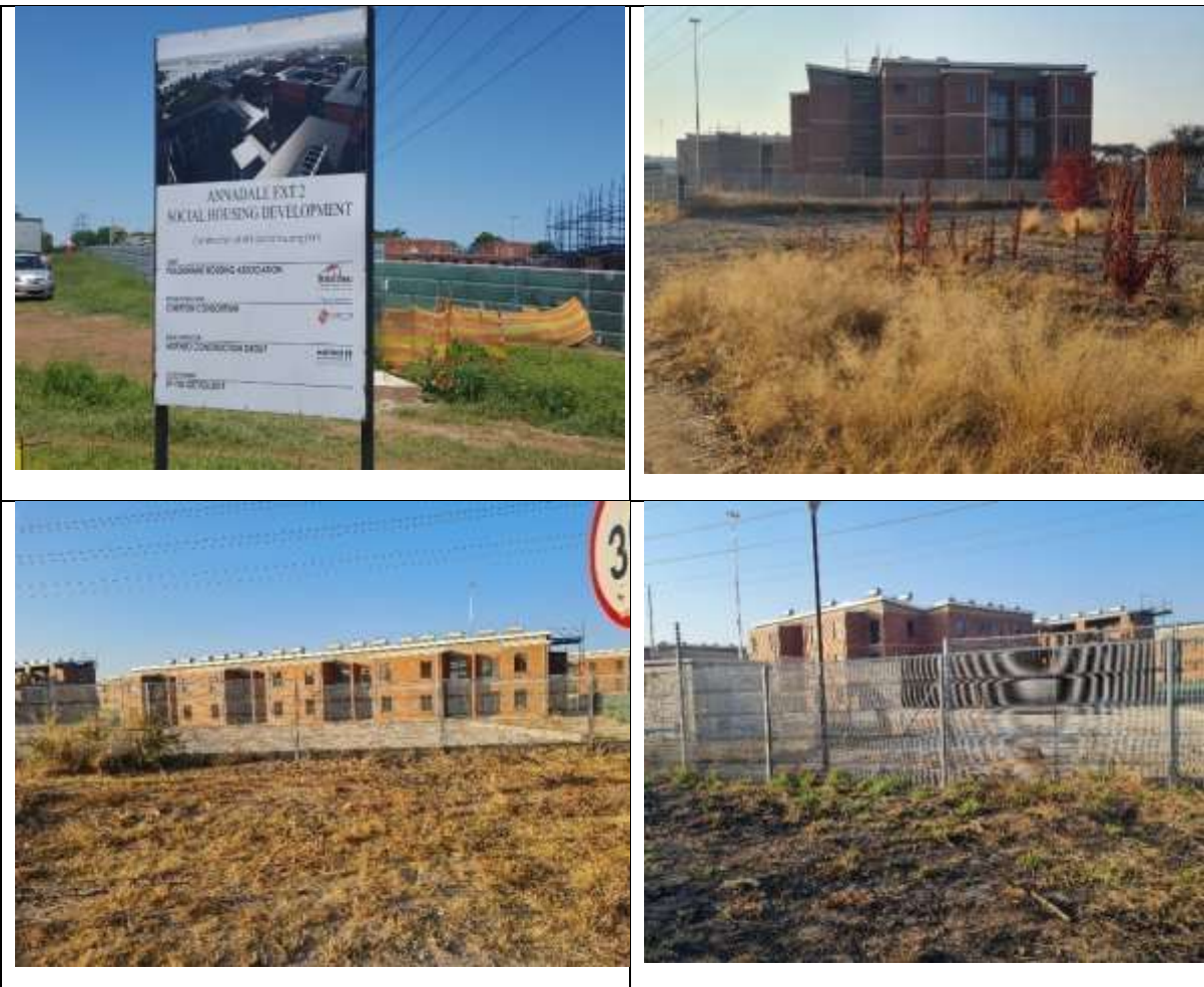
Construction of Ga-Rena Phase 2
