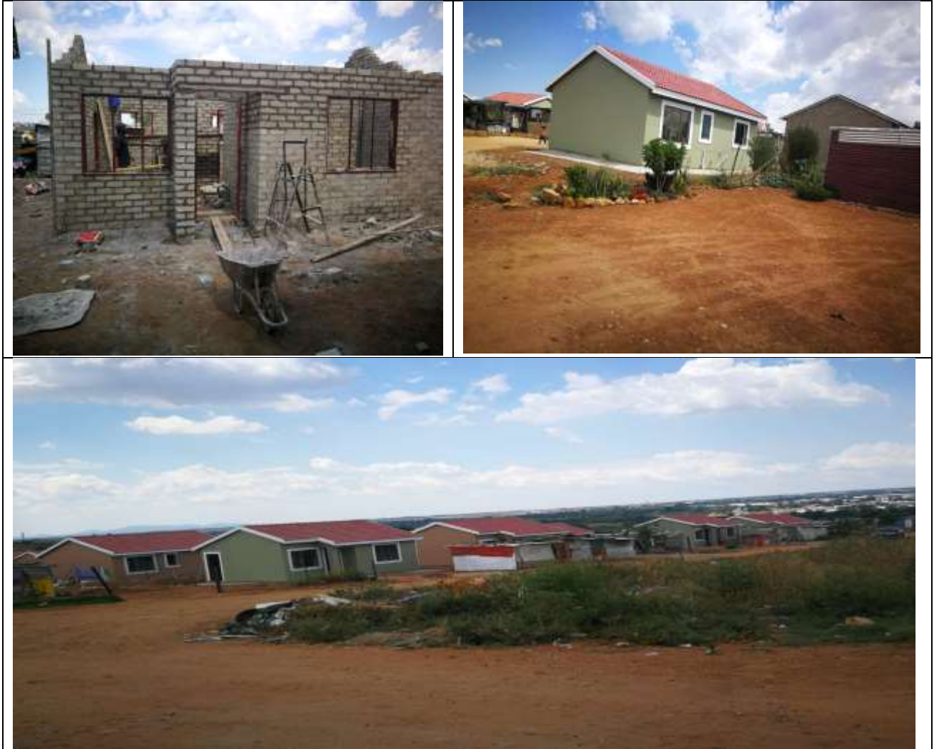
RDP Construction at ward 08
